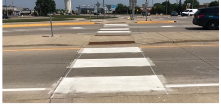
Figure 7. Motorcycle-friendly crosswalk markings.
