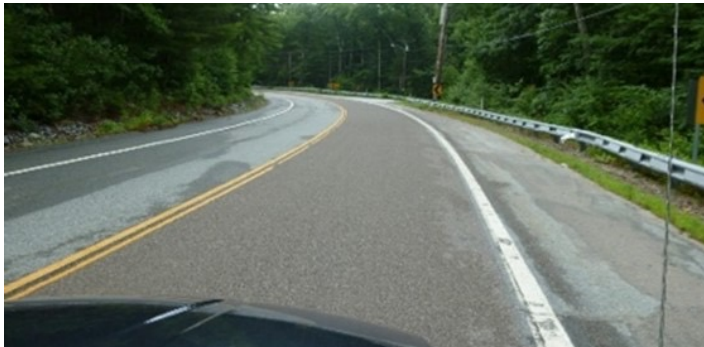
Figure 12. High-friction surface treatment installation
